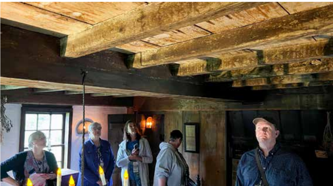
...with a well-built beamed ceiling,...
